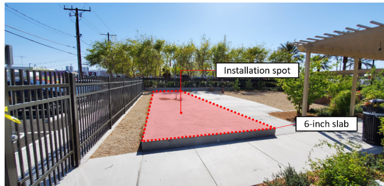
Figure 4. Modular house job site installation spot
