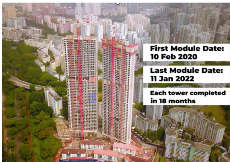
Fig.4. Photo of the completed towers
